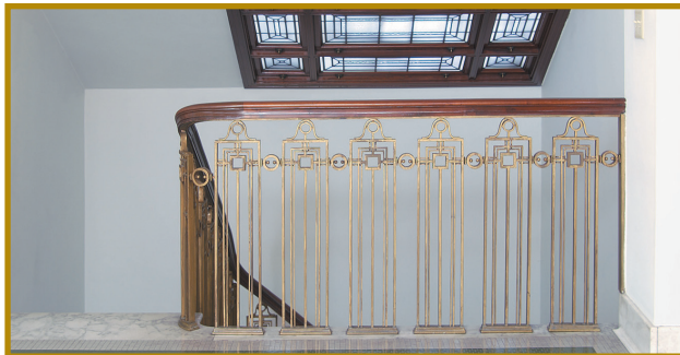
Decorative staircase metal work.
